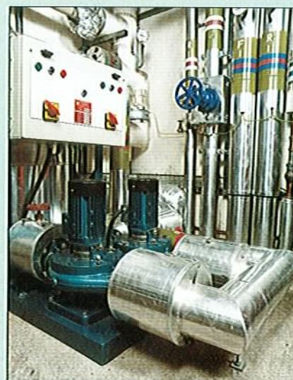
Three JM(UK) sets in production for a soap factory in Indonesia. Because of the damp climate the control panels included special heaters.
